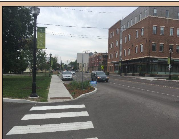
Completion of the first phase of the Federal Street Multimodal Connector.
